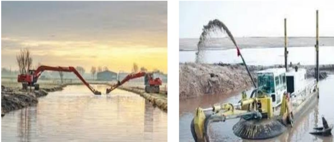
Figure 7: Dredging and widening of water channels for navigation
