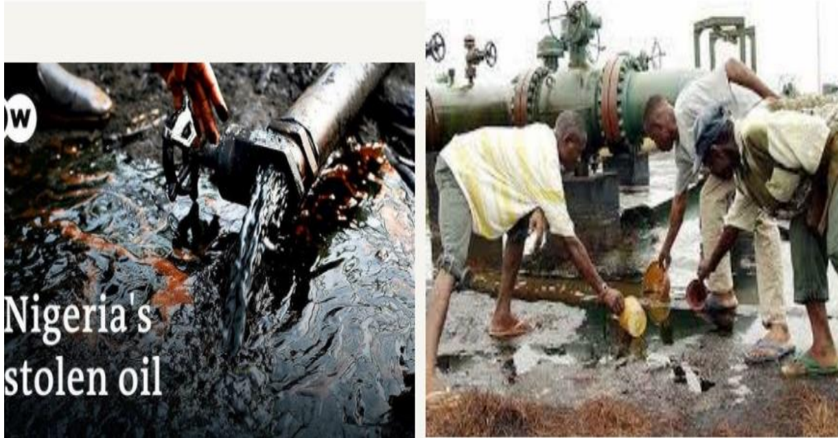
Figure 4; Oil pipeline vandalism and stealing
