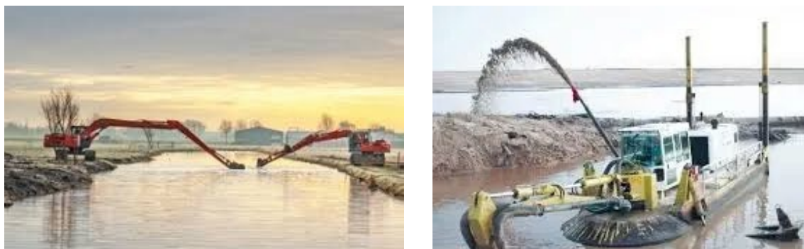
Figure 7: Dredging and widening of water channels for navigation
